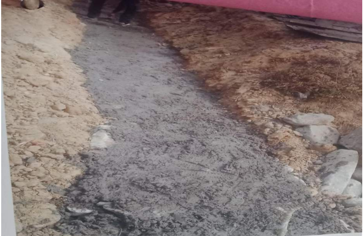
Construction of Hume Pipe Bed
