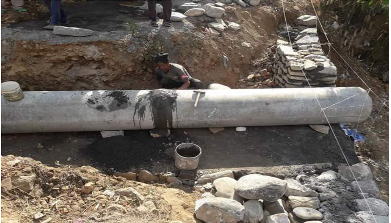
Hume Pipe Laying (Permanently)
