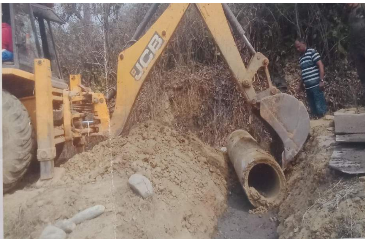
Hume Pipe Laying
